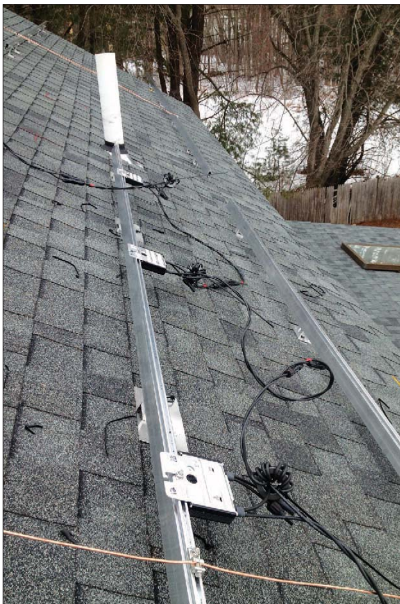
Figure 6 — The chokes from Figure 2, as well as the twisted wire transmission cables can be seen between two of the aluminum support rails before solar panels were installed.
